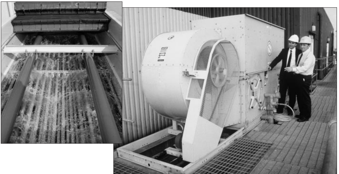
Figure 25 Evaporative condenser
