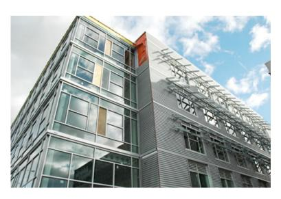
Office building in Seattle, Washington, USA designed by Weber & Thomson requires no air-conditioning. The building has green-tinted glass shades (or sunglasses) that shield windows from heat, while still allowing light into the building. Heat-reflective coating on the windows also reduce temperatures. The 40,000 square foot structure has a central courtyard, which allows cross breezes to enter all parts of the building, and allows more natural light into the building.<sup>66</sup>
