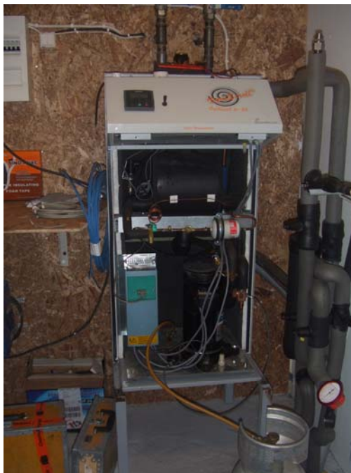
Fig. 27: Heat Pump Test Rig
