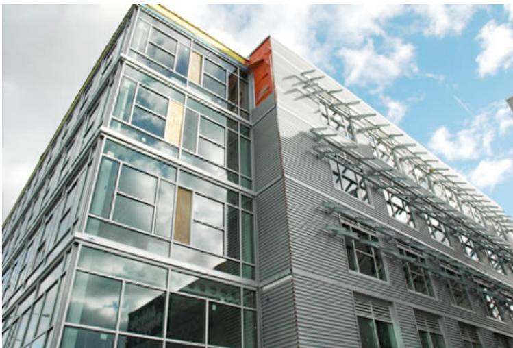
Office building in Seattle, Washington, USA designed by Weber & Thomson requires no air-conditioning. The building has green-tinted glass shades (or sunglasses) that shield windows from heat, while still allowing light into the building. Heat-reflective coating on the windows also reduce temperatures. The 40,000 square foot structure has a central courtyard, which allows cross breezes to enter all parts of the building, and allows more natural light into the building.<sup>66</sup>
