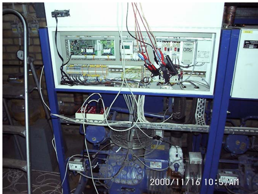
Figure 30b. SQD System Machine Room
