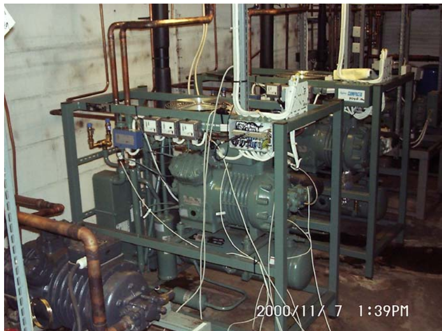
Figure 29b. DX System Machine Room
